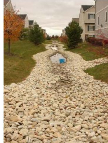
Rock-lined swale in residential complex
