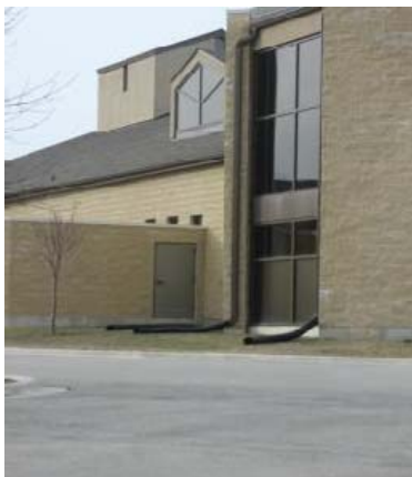
Roof runoff retrofit opportunity
